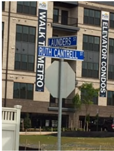
Pulte Condominiums under construction west of subject
