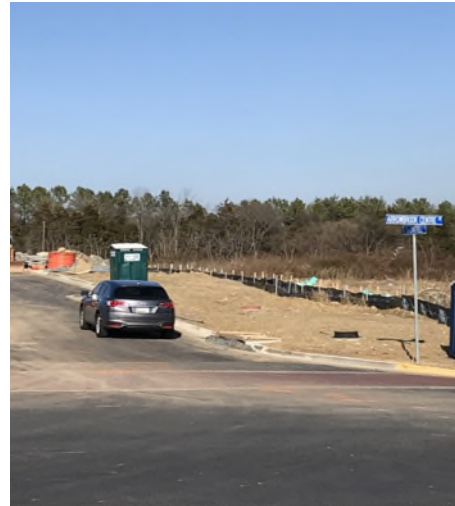
Looking northeast at site from Arrowbrook Centre Drive
