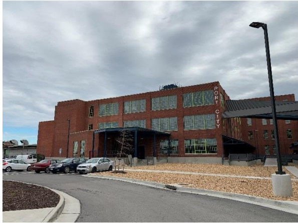
Port City Apartments
