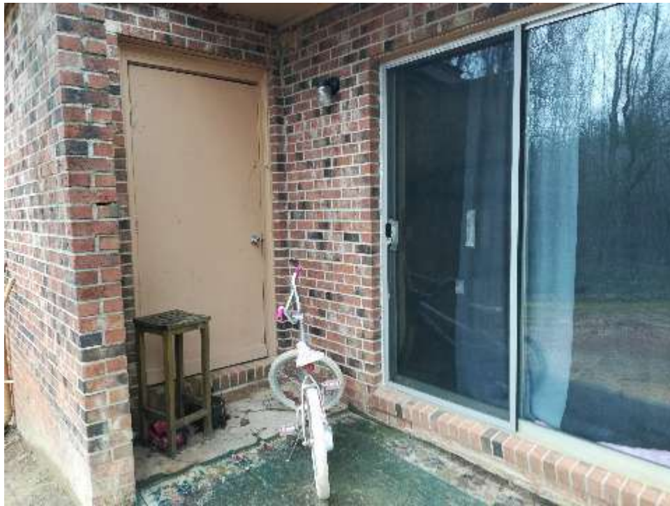
View of Typical Patio and Extra Storage
