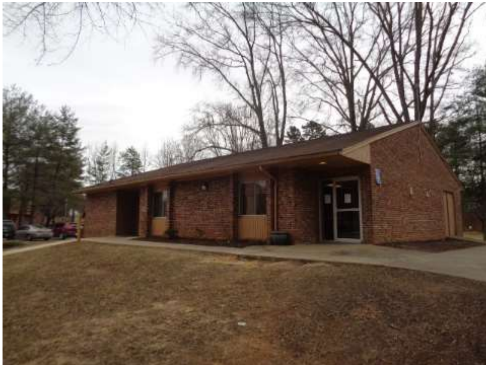
View of Accessory Building - Exterior
