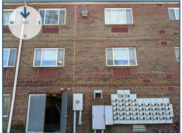
View of site from the north
