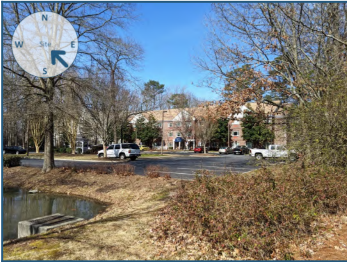
View of site from the southeast
