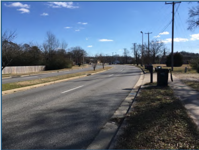
Streetscape: Southeast view of Warwick Road
