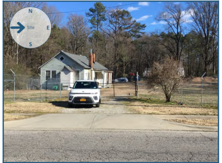
View of site from the west
