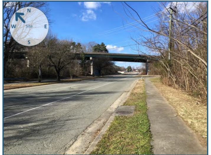
Northwest view from site
