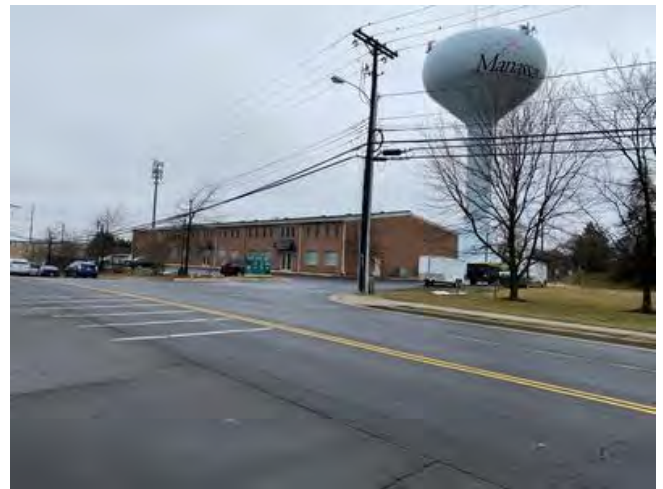
Commercial uses located south of Subject
