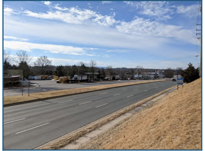
Streetscape: Northeast view of Seminole Trail (U.S. Highway 29)
