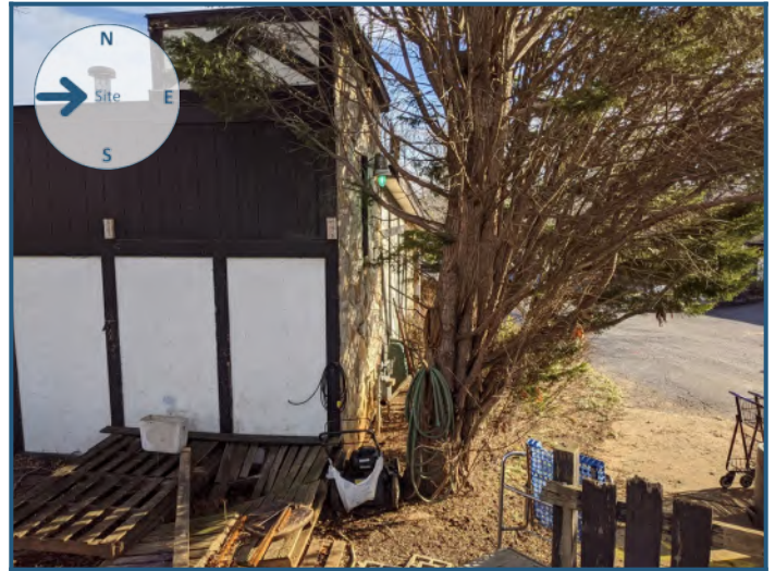
View of site from the west
