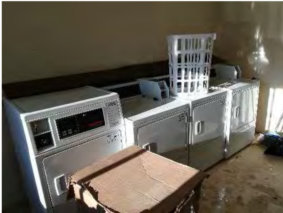
View of Laundry Facility
