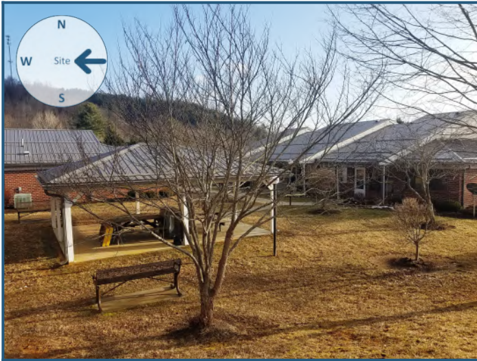
View of site from the east
