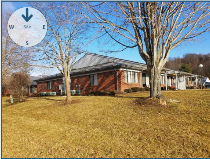
View of site from the north
