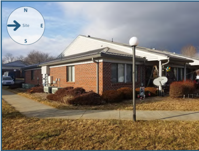
View of site from the west
