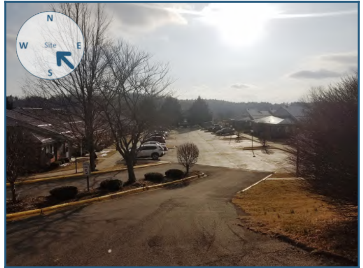
View of site from the southeast
