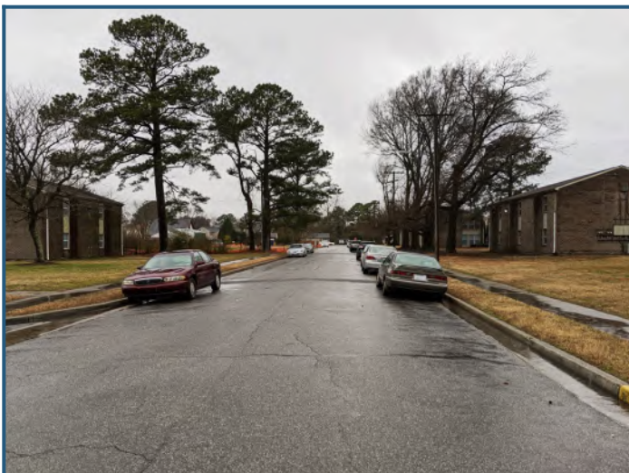
Streetscape: West view of Bird Lane
