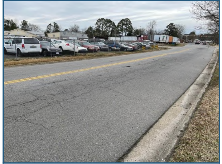
Streetscape: North view of Deep Creek Boulevard
