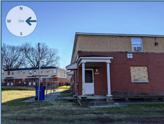
View of site from the east
