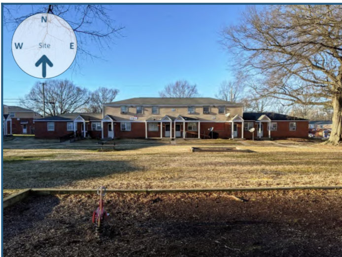
View of site from the south
