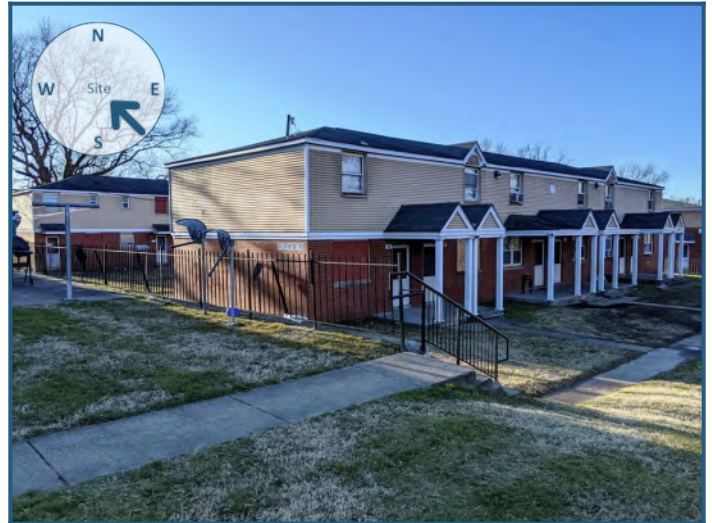
View of site from the southeast
