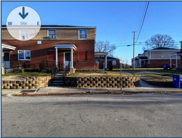
View of site from the north
