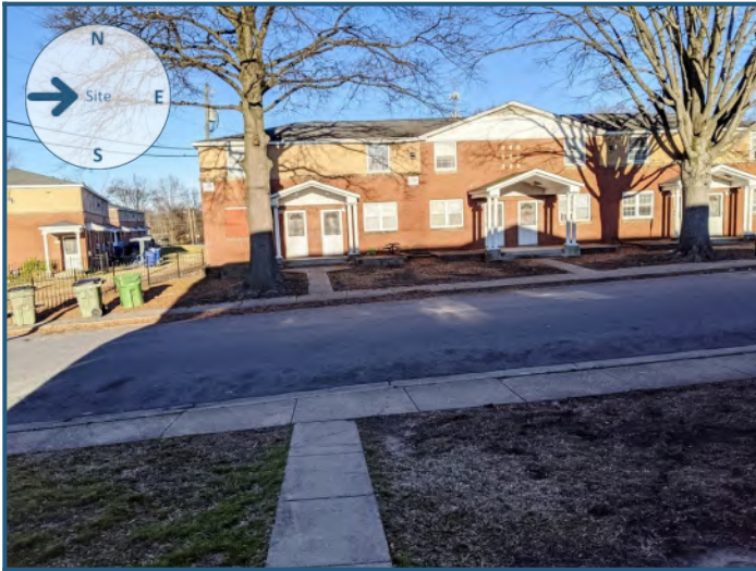
View of site from the west
