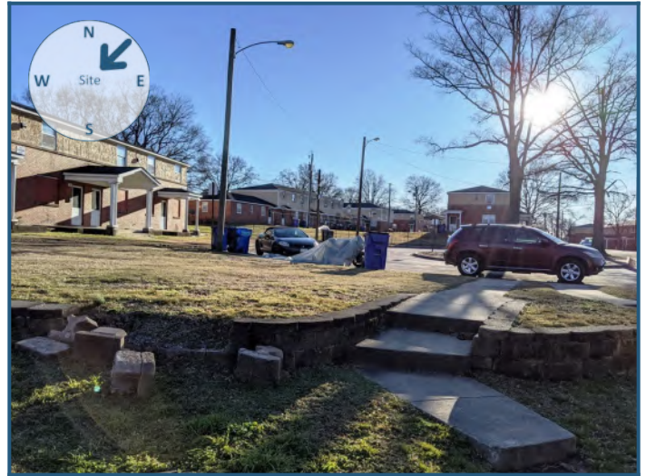
View of site from the northeast
