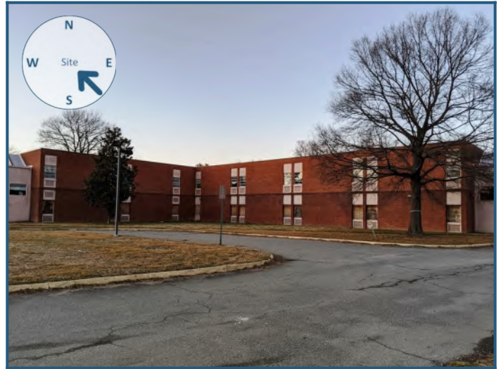
View of site from the southeast
