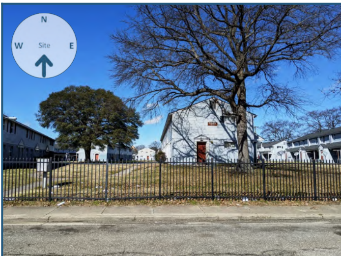
View of site from the south
