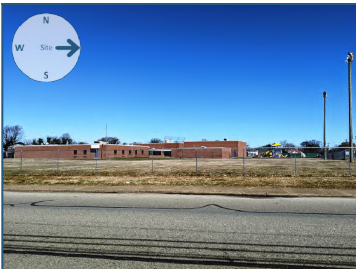
East view from site
