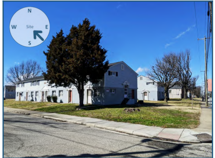
View of site from the southeast
