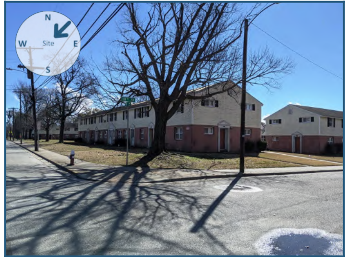
View of site from the northeast
