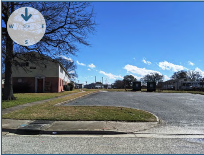
View of site from the north
