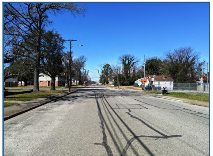
Streetscape: South view of Ivy Avenue
