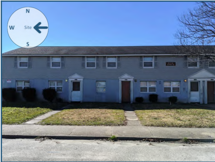
View of site from the east
