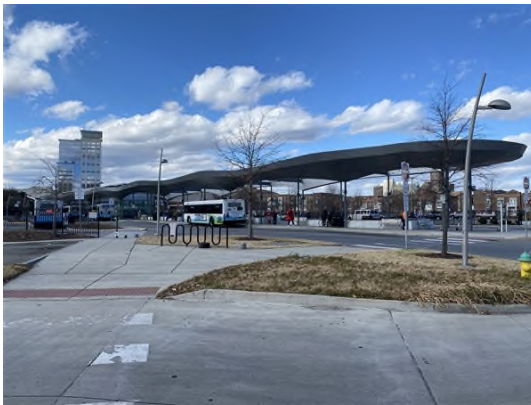
Transit Center northwest of subject site
