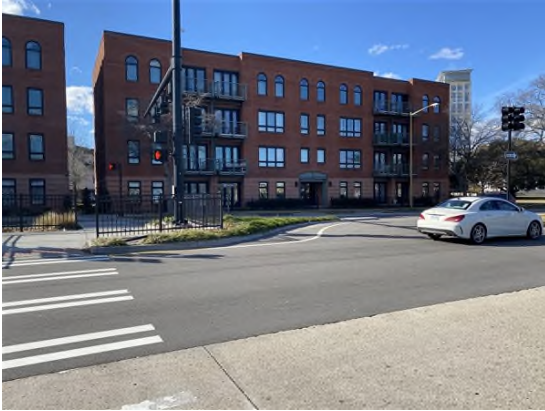
Condo community west of site
