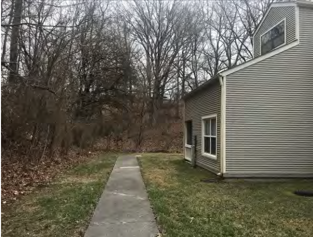
TYPICAL WALKWAY/UNIT ENTRANCE
