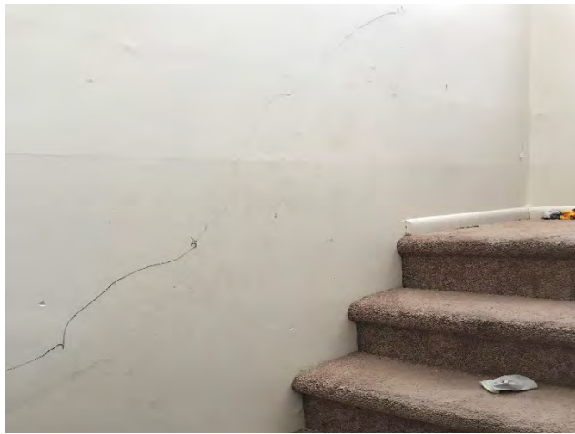
TYPICAL STAIRWAY (TH)
