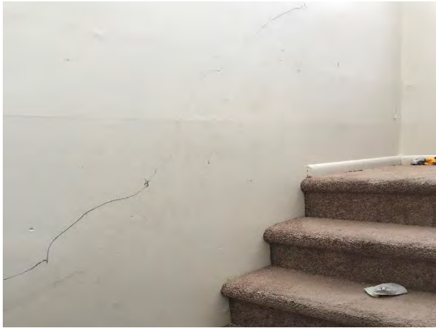
TYPICAL STAIRWAY (TH)
