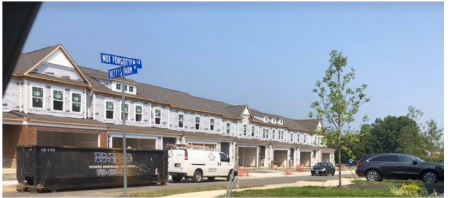
Homes Under Construction Near Site
