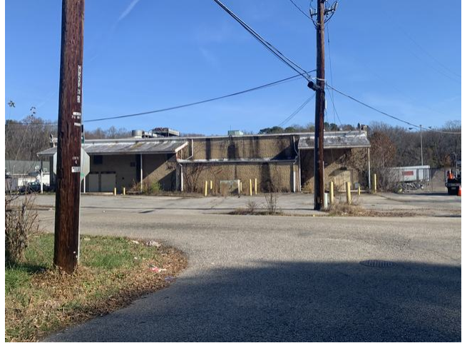
Vacant commercial building north of Subject
