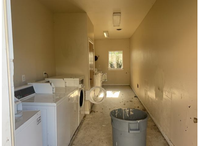
Central laundry facility
