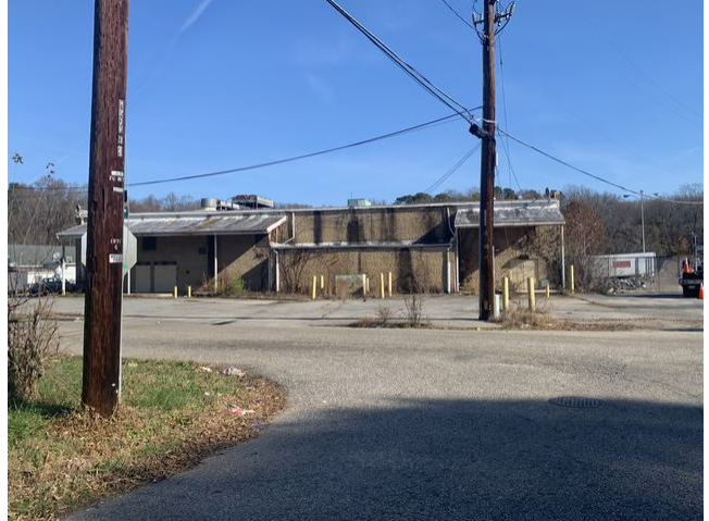
Vacant commercial building north of Subject
