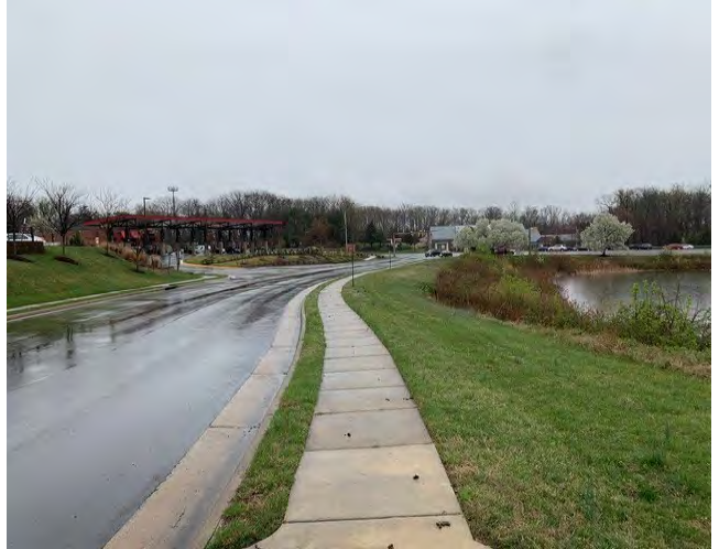
VIEW FACING SOUTH ALONG NOBLE POND WAY
