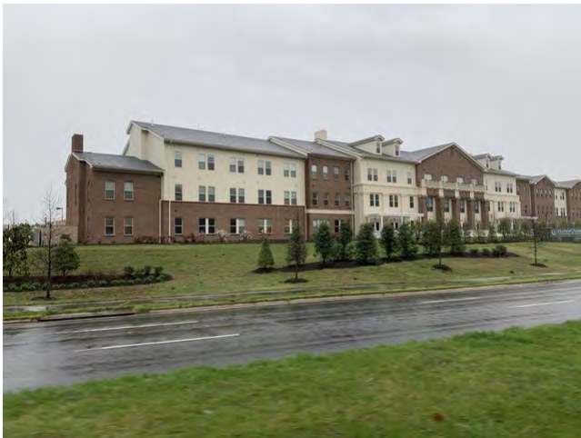
ASSISTED-LIVING FACILITY ADJACENT TO SUBJECT SITE
