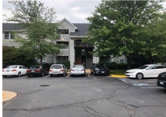
Exterior - Dulles, Phase II
