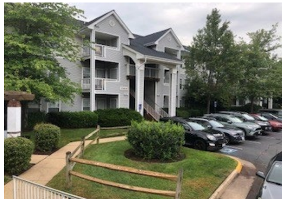
Exterior - Dulles, Phase II
