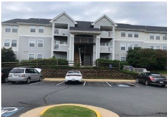
Exterior - Dulles, Phase II
