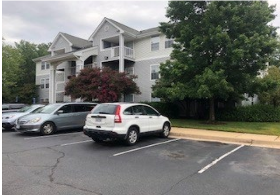
Exterior - Dulles, Phase II
