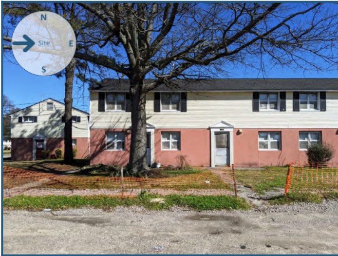
View of site from the west
