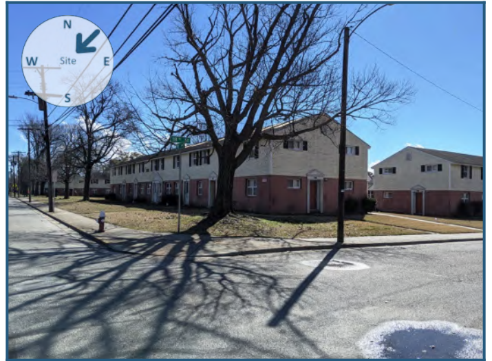
View of site from the northeast
