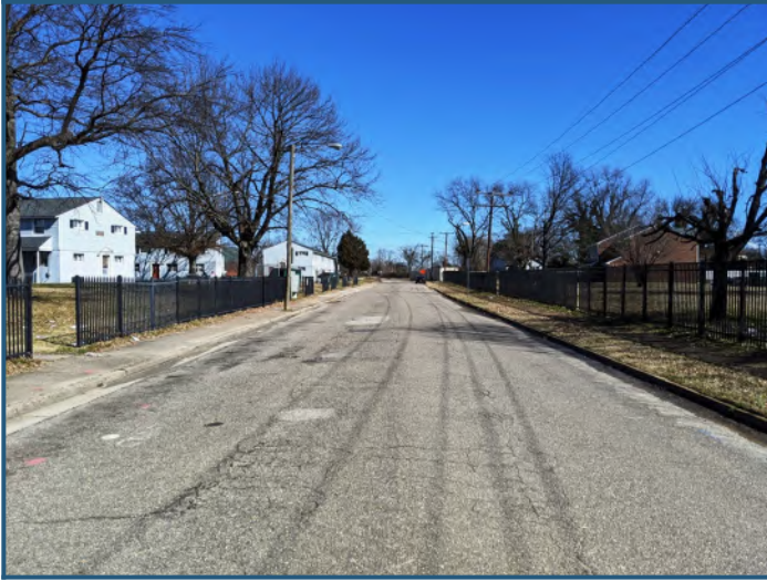
Streetscape: East view of 12th Street
