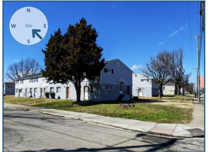
View of site from the southeast
