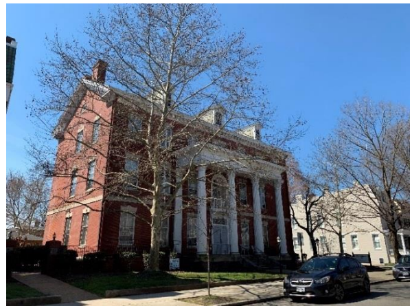
Columns on Grove
