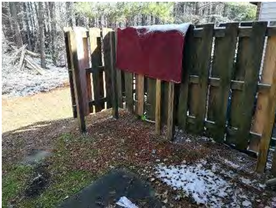
View of Typical Patio
