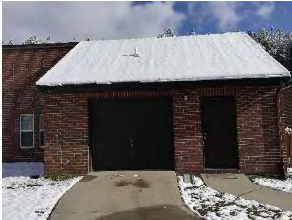
View of Maintenance Area
