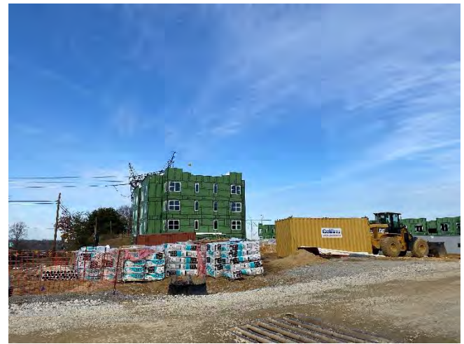
Under construction Phase I of the Subject (outside scope of report)
