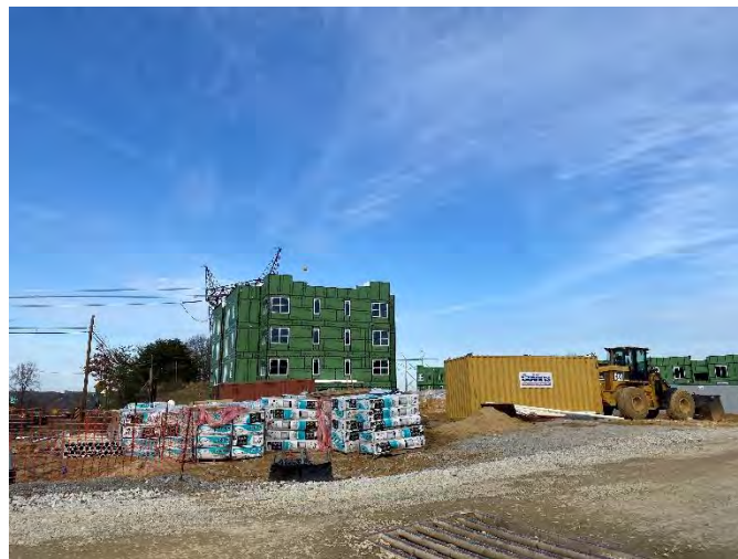
LIHTC development (part of the Townsquare at Dumfries development)
