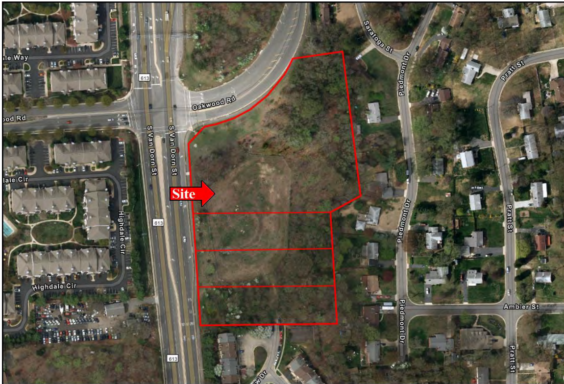
Northern Aerial of Oakwood South Nine Site
