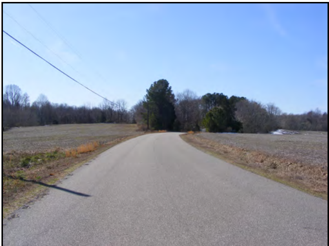
View south on Oakland Drive, at site
