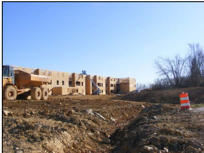
View from site to second phase
