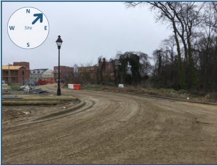
Northeast view from site
