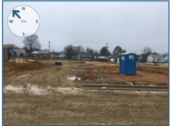
Northwest view from site
