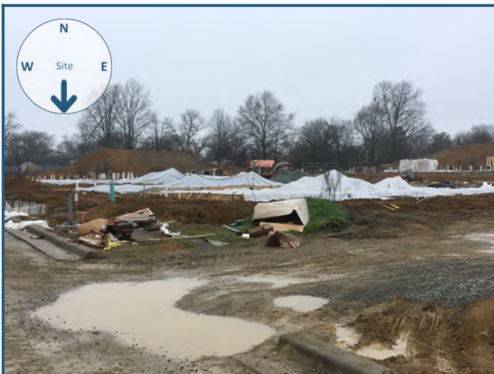
South view from site
