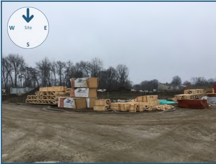
View of site from the north
