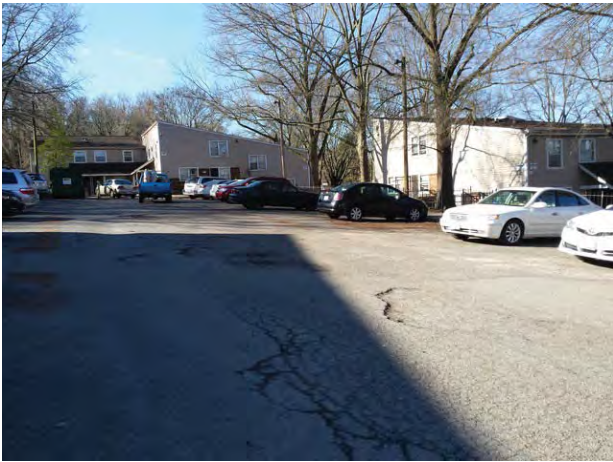
Subject parking area
