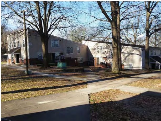
Typical Subject building
