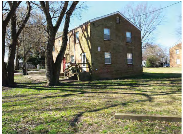
Typical Subject building
