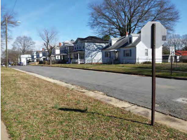
Single-family homes along West 33 rd Street to the east of Subject
