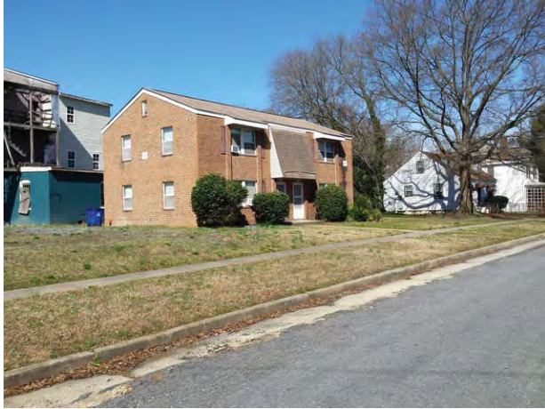
Subject from West 33 rd Street looking northwest
