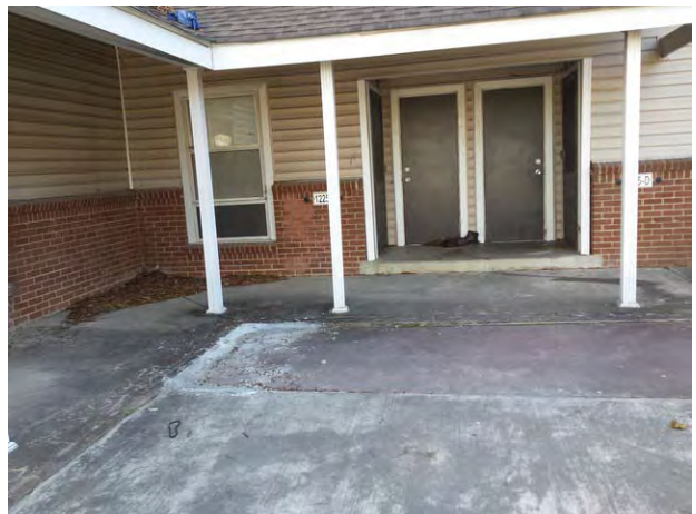
Typical unit entrance area
