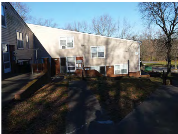
Typical Subject building
