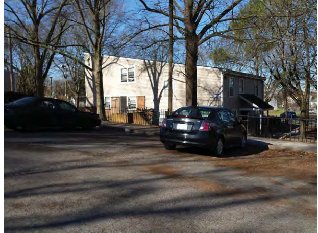
Typical Subject building from parking area
