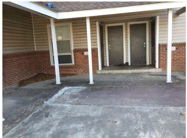
Typical unit entrance area
