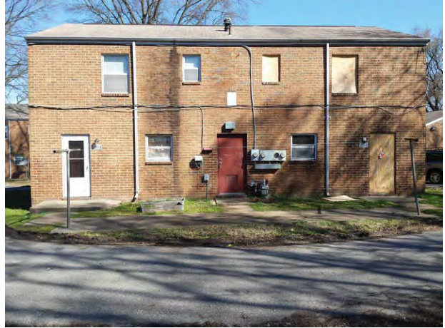
Rear of typical Subject building
