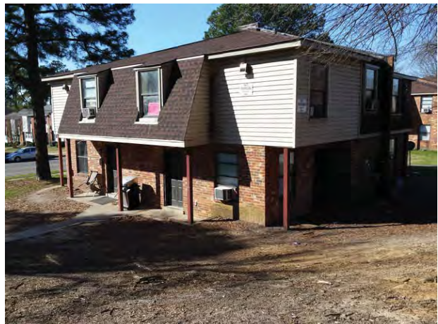
Typical Subject building
