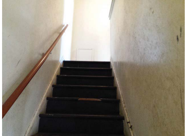
Typical interior stairway – vacant unit
