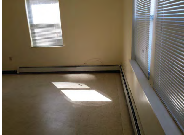
Typical living area – vacant unit
