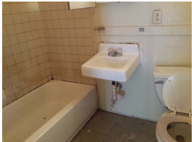
Typical bathroom – vacant unit
