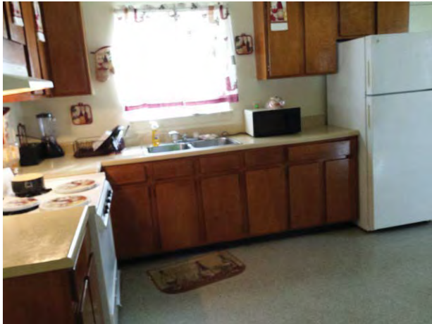
Typical kitchen – occupied unit
