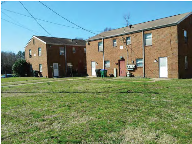
Rear of typical Subject buildings
