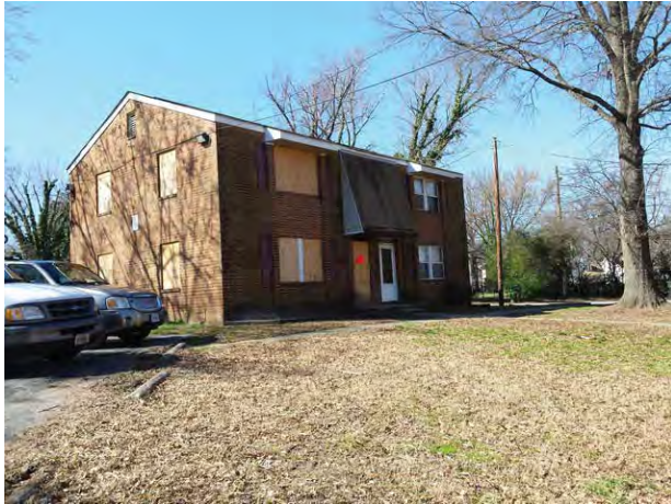
Subject building with boarded-up unit and parking area
