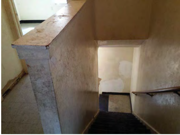
Typical interior stairway - vacant unit
