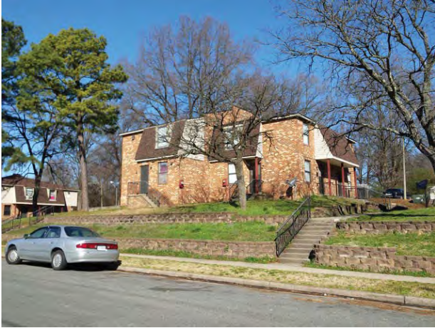
Typical Subject building from Afton Avenue looking north
