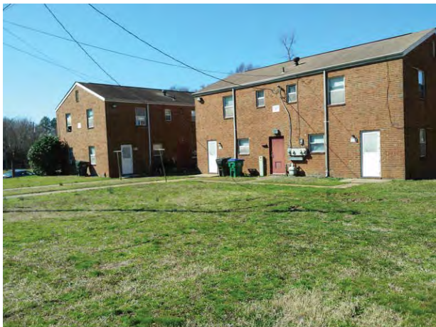
Rear of typical Subject buildings
