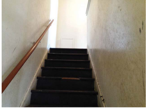
Typical interior stairway - vacant unit
