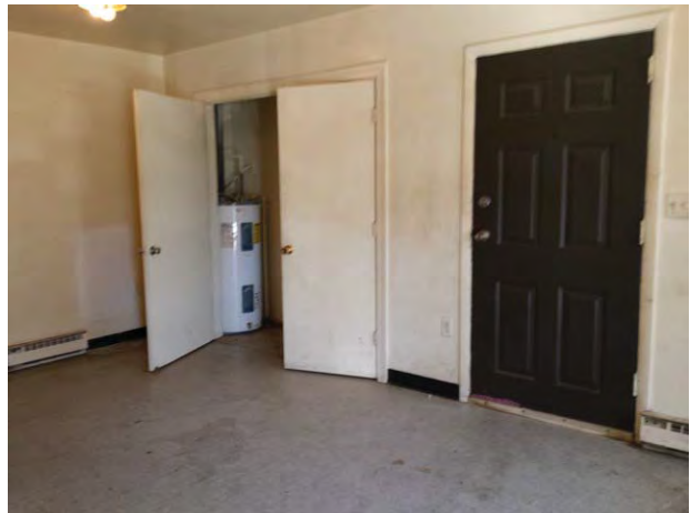
Typical living area – vacant unit
