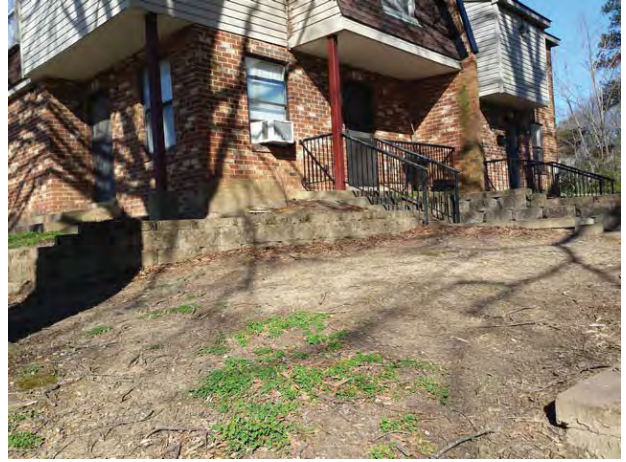
Typical building entrance area
