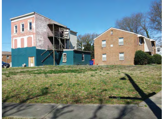
Typical Subject building (right side of photo) from Moody Avenue looking north
