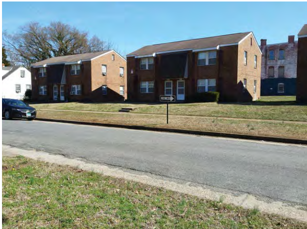
Subject buildings from West 34 th Street looking east
