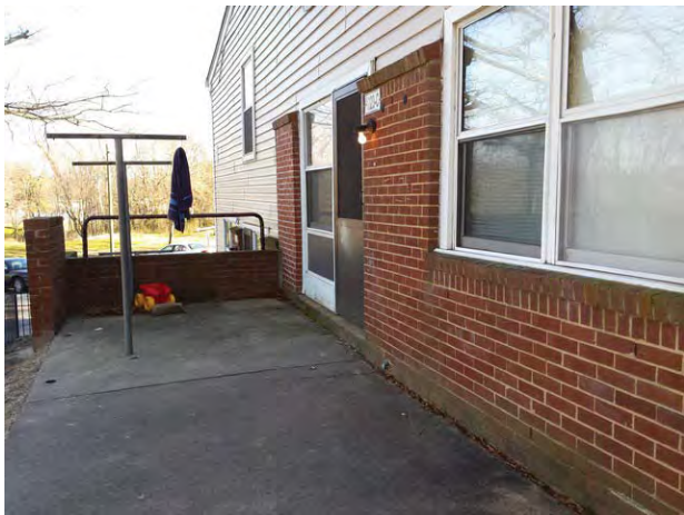
Typical patio area
