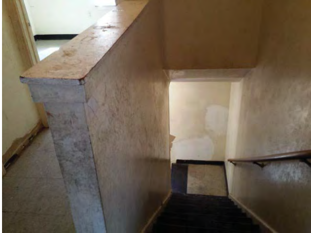
Typical interior stairway – vacant unit
