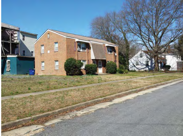
Subject from West 33 rd Street looking northwest
