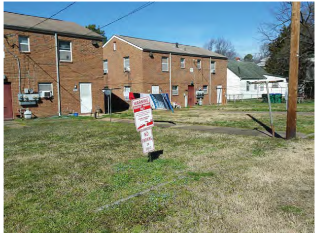
Rear of typical Subject buildings
