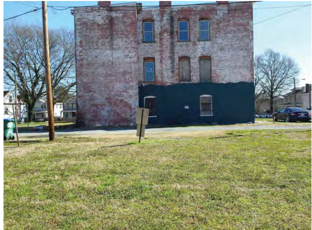
Alternative view of vacant building (under rehabilitation to the rear of Subject site)
