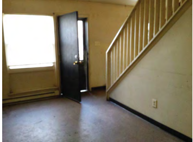
Typical living area – vacant unit
