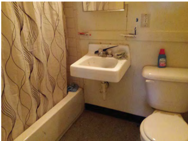
Typical bathroom – occupied unit
