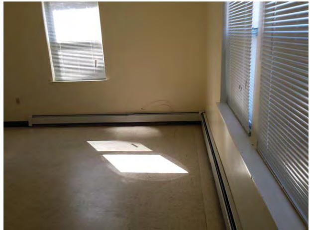
Typical living area – vacant unit
