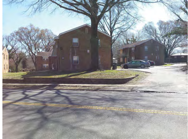
Subject from Bainbridge Street looking southeast
