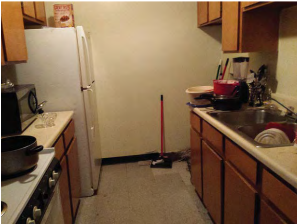
Typical kitchen – occupied unit
