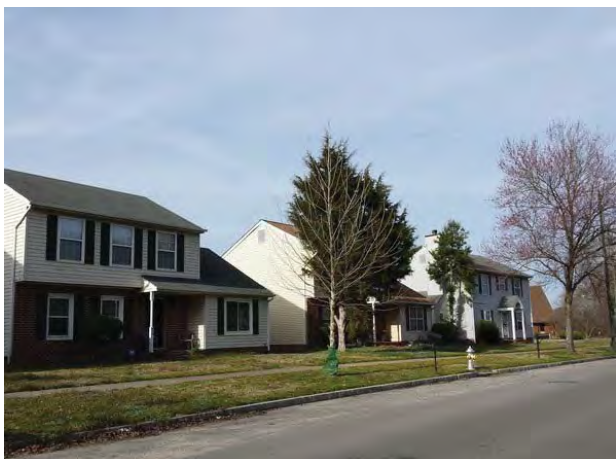
Single-family home along Admiral Gravely Boulevard to the west of Subject
