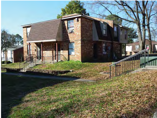
Typical Subject building
