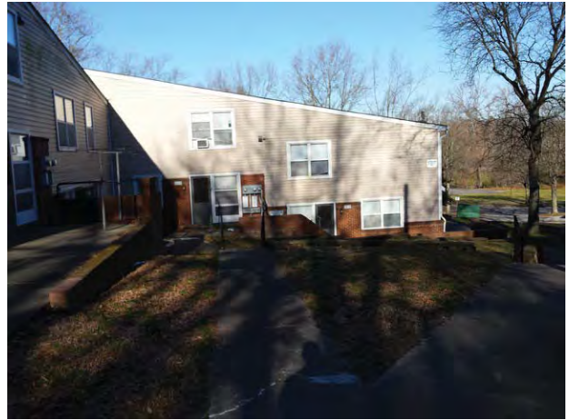
Typical Subject building
