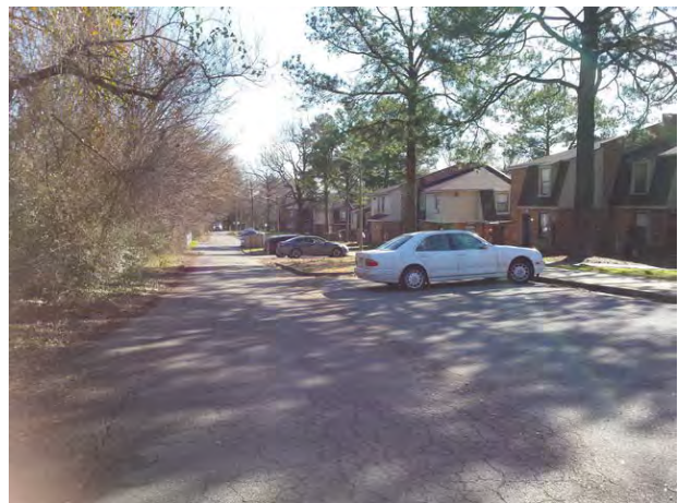
View of rear parking area looking east
