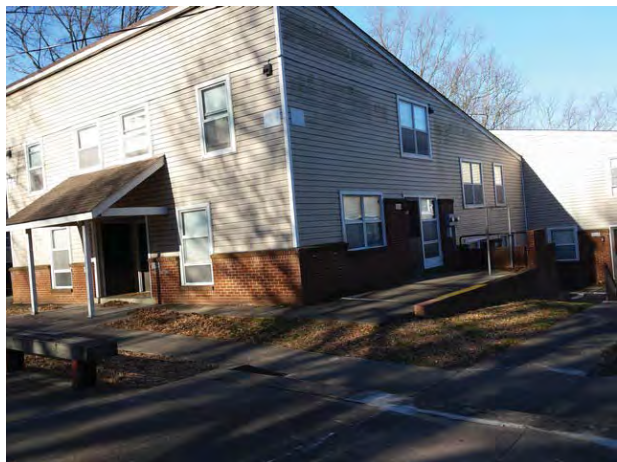
Typical Subject building
