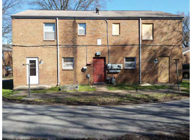
Rear of typical Subject building
