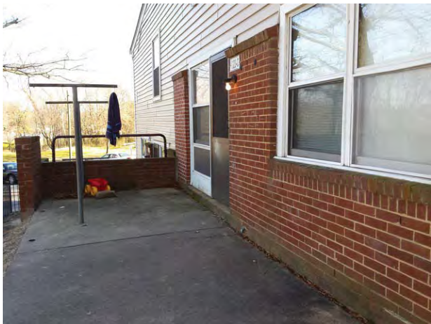
Typical patio area
