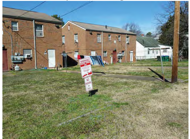
Rear of typical Subject buildings
