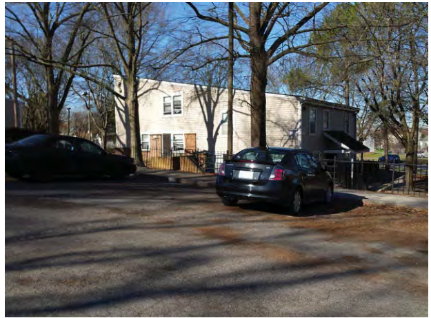
Typical Subject building from parking area
