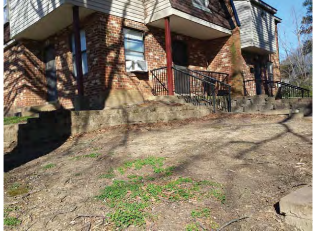
Typical building entrance area
