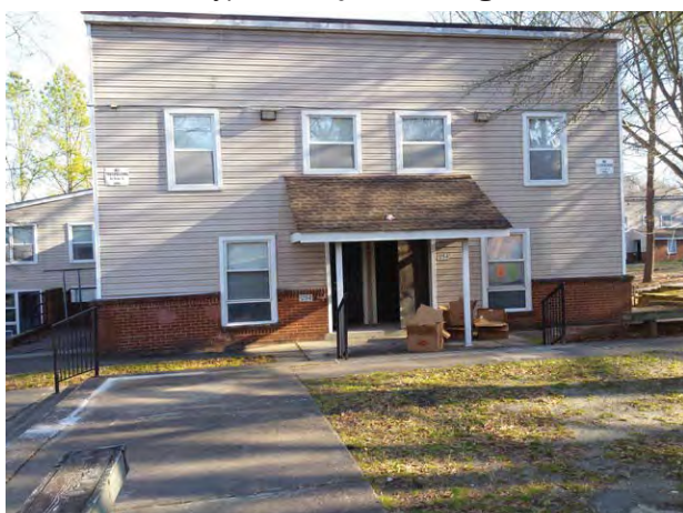
Typical Subject building
