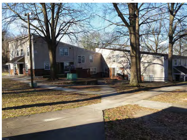
Typical Subject building
