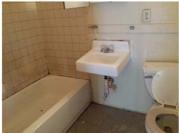
Typical bathroom - vacant unit
