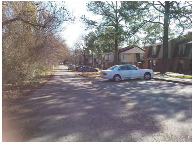
View of rear parking area looking east
