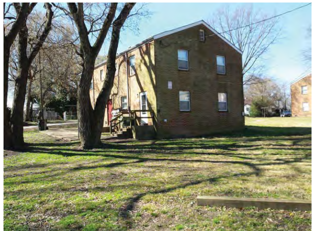
Typical Subject building
