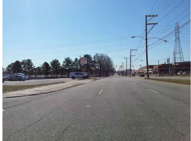
U.S. Route 1 looking south from Afton Avenue
