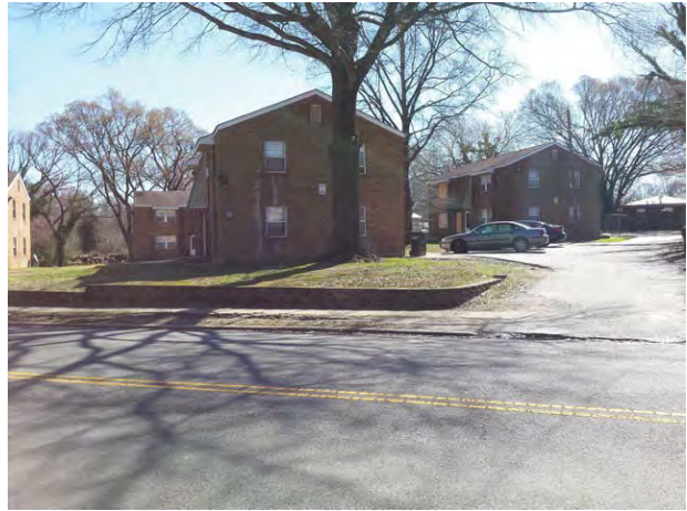
Subject from Bainbridge Street looking southeast
