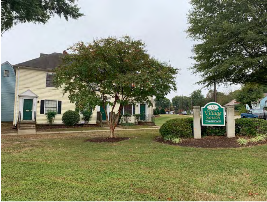
Village South Townhomes (Holly Springs) – Holly Springs Road View, Area Probe LLC
