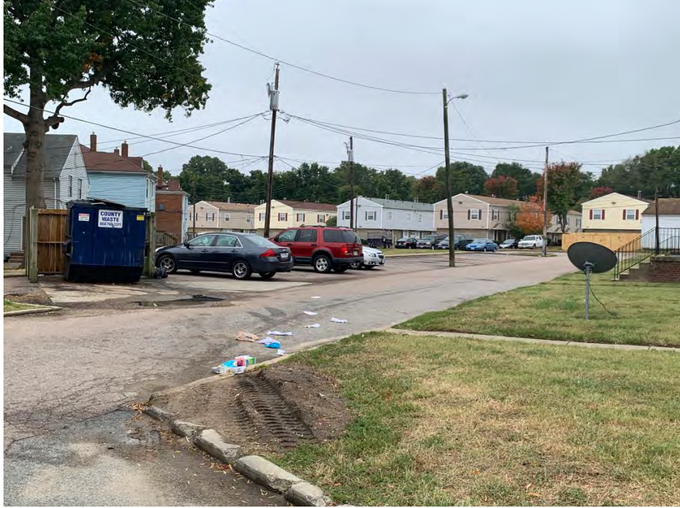
Village South Townhomes – Parking Lot, Holly Springs, Area Probe LLC
