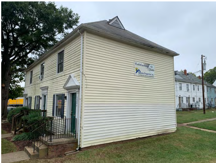
Village South Townhomes – Maury Street View, Area Probe LLC
