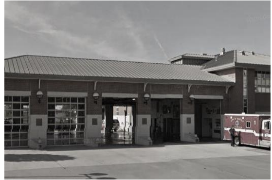
Fire station west of site
