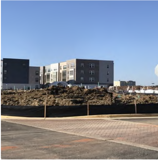
Pulte Condominiums under construction west of subject
