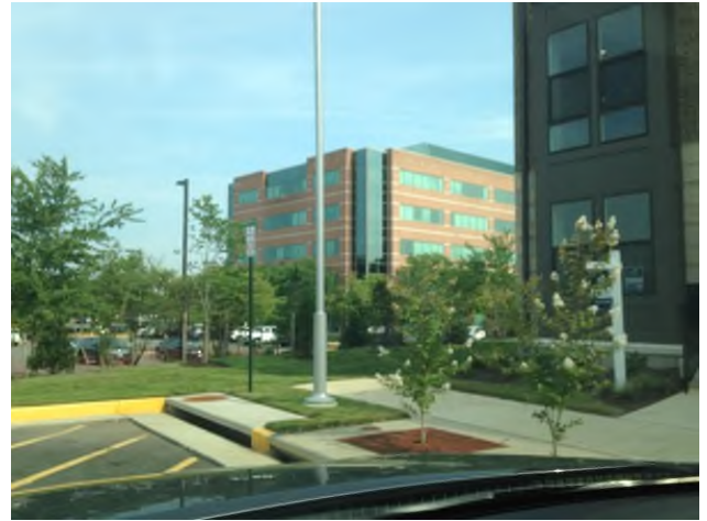
Office building on western portion of Arrowbrook Centre campus
