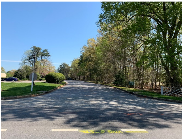
Site Access from Pocahontas Trail
