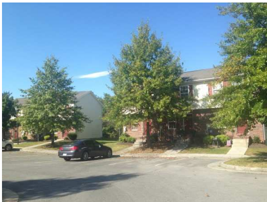
General occupancy multifamily community east of subject site
