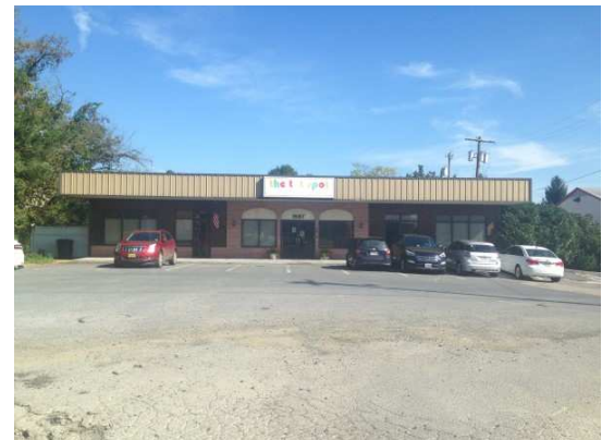
Strip retail center east of subject along Senseny Road
