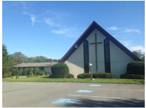
Improvements on site expected to be demolished
