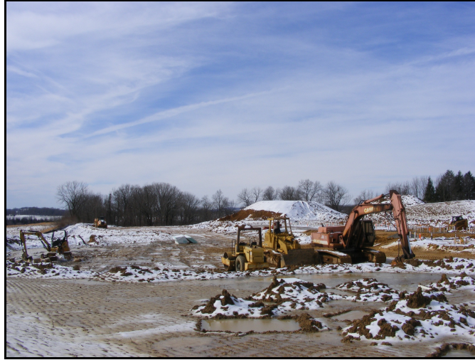
Ongoing construction, Phase I
