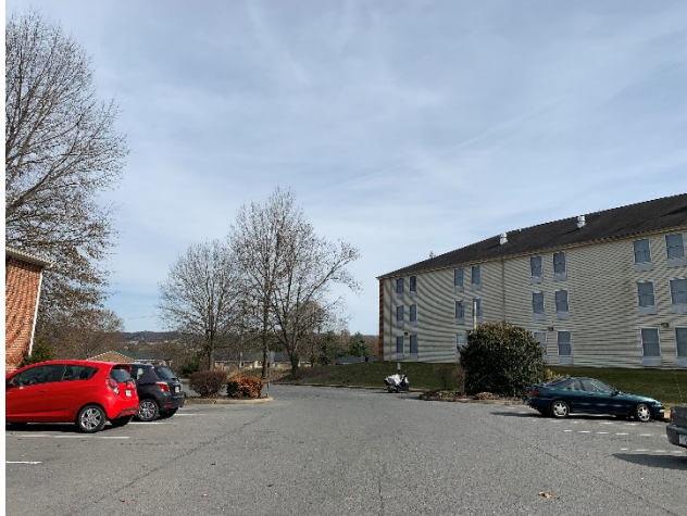
Typical Parking Area
