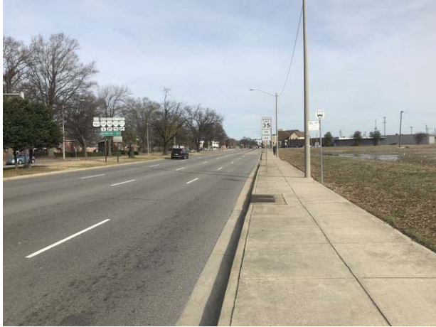
View north along Tidewater Drive
