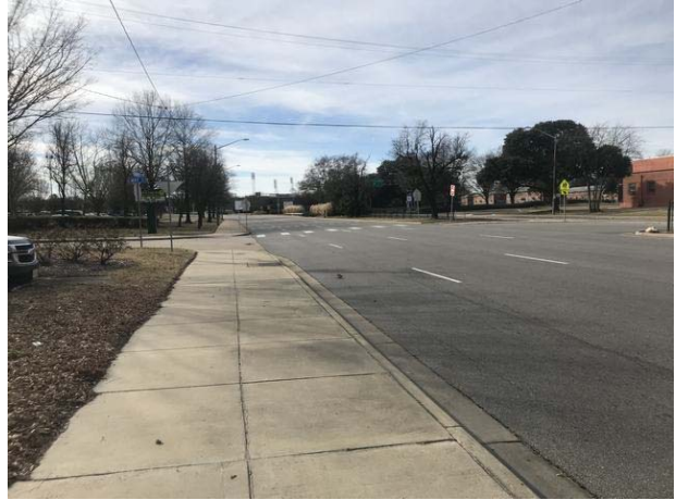
View south along Tidewater Drive
