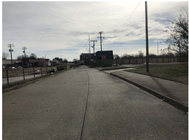
View east along E. Brambleton Avenue
