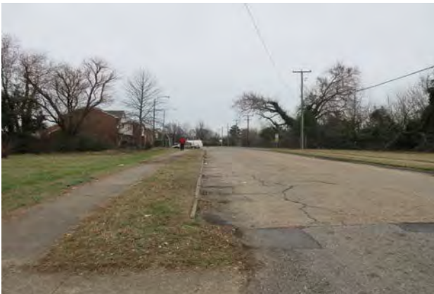
Looking East From Entrance
