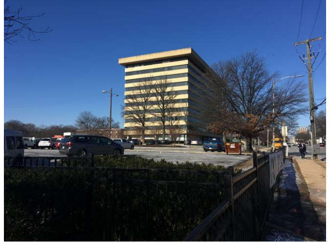
Office building and parking lot east of Subject
