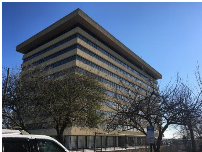
Office building east of the Subject
