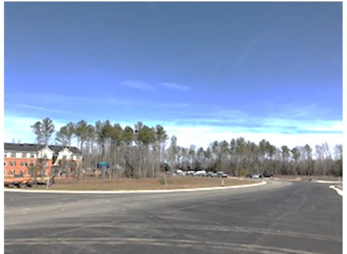
Second View North to King William Manor Site
