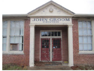
3. BLDG 1 - ORIGINAL ENTRANCE
