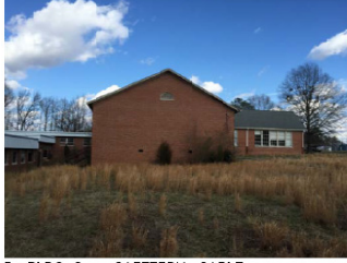
5. BLDG 2 - CAFETERIA GABLE
