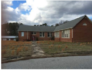
1. BLDG 1-ORIGINAL SCHOOL AND CAFETERIA
