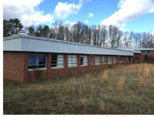
6. BLDG 3 - REAR ADDITION (1959)
