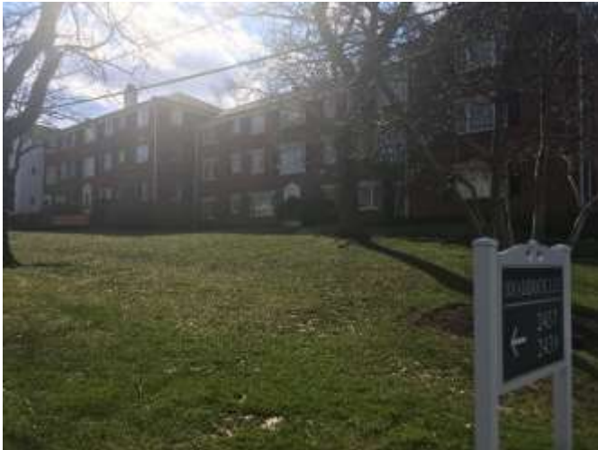
Braddock Lee Apartments to the west of Subject site
