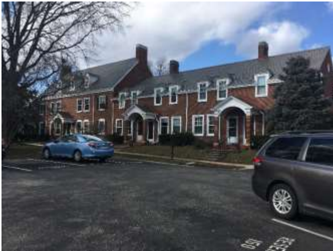
Fairlington Mews Condominiums northeast of the Subject site
