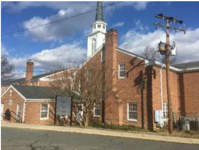
View looking east from the Subject site
