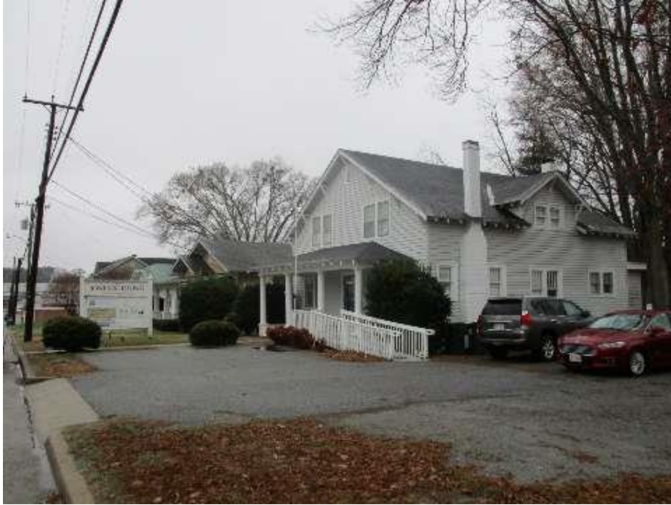
View to the North
