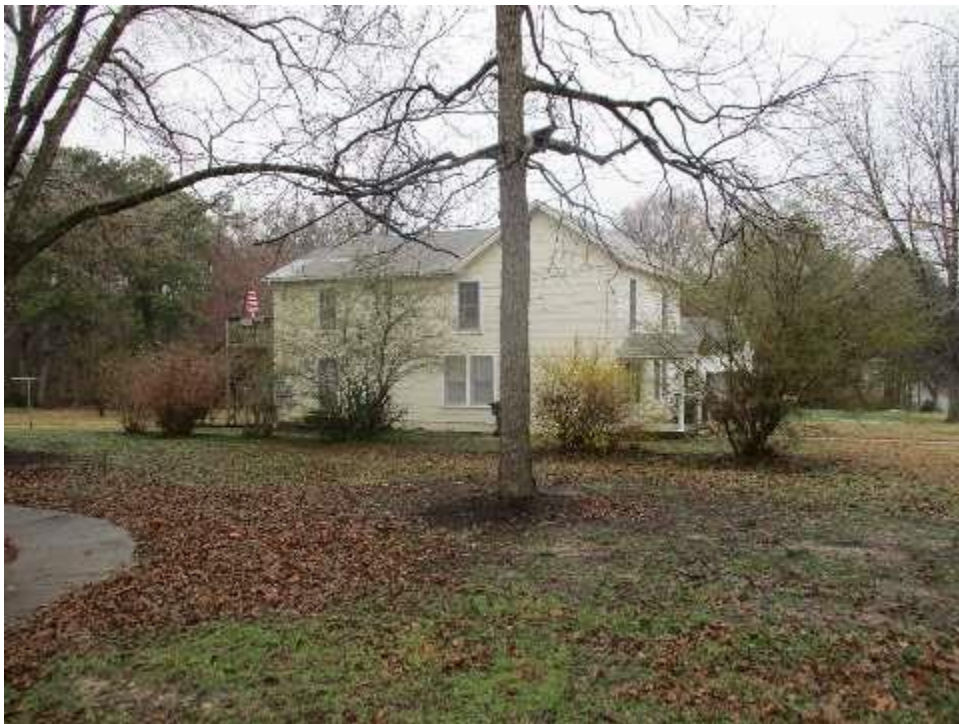
View to the South
