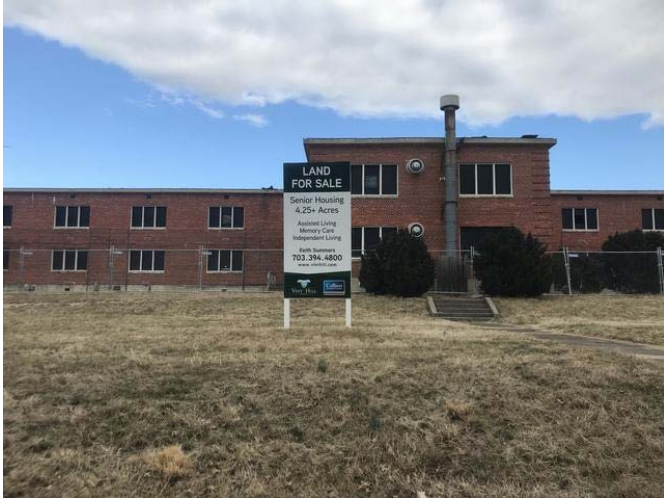
View southwest from the Subject site
