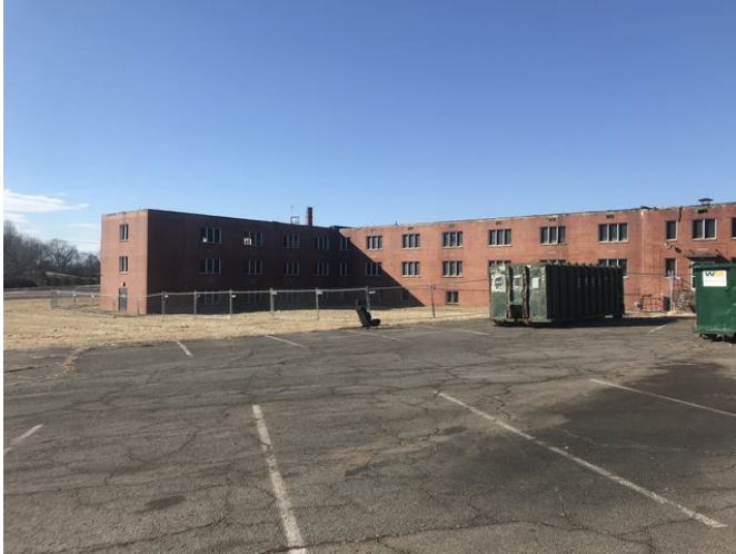
View south of the Subject site
