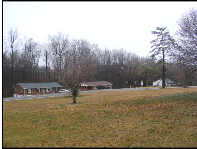
View from front of school
