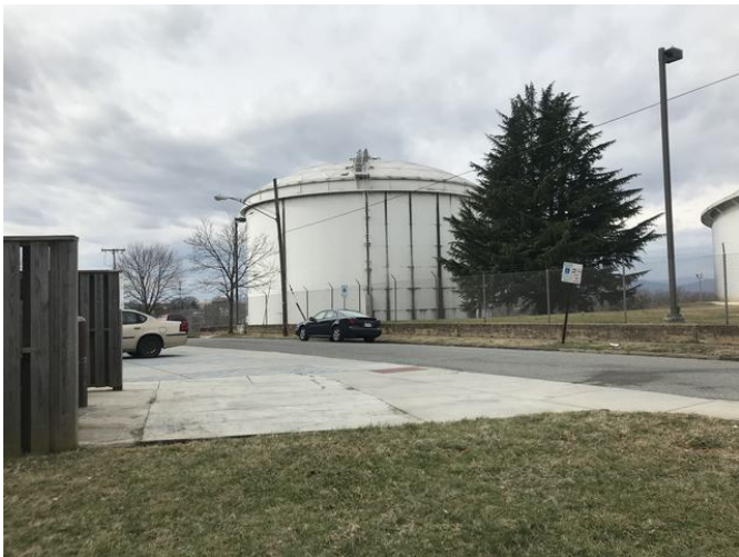
Water treatment facility north of the Subject
