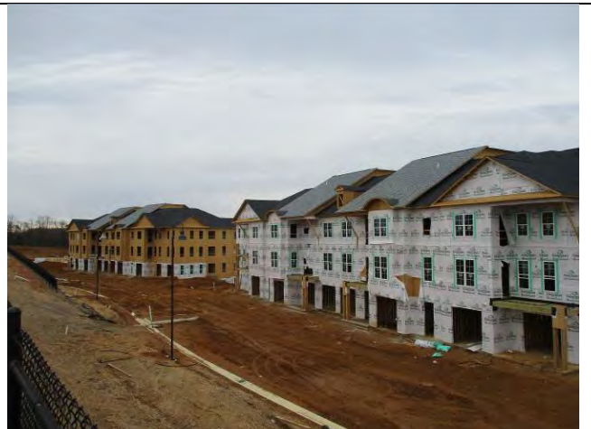
THE ALLURE AT JEFFERSON - MULTIFAMILY USE UNDER CONSTRUCTION NORTH OF SUBJECT
