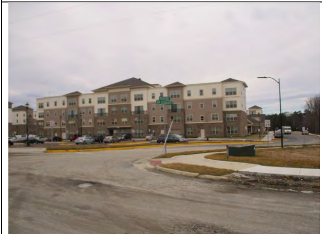
ORCHARD RIDGE AT JACKSON VILLAGE PHASE II – MULTIFAMILY USE SOUTH OF SUBJECT
