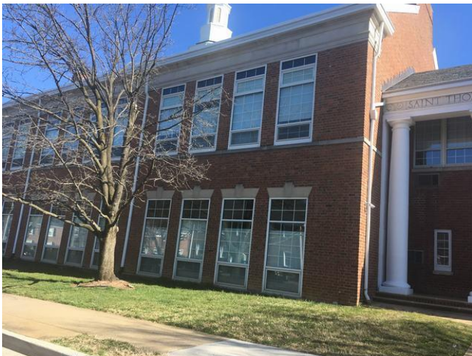
St. Thomas More School northeast of the Subject site
