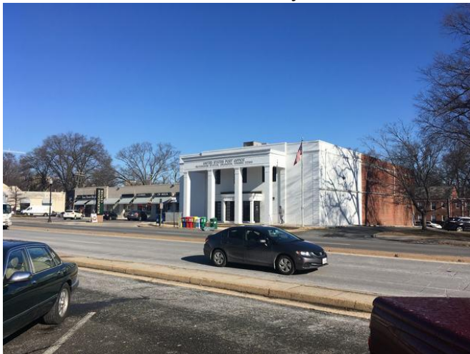
Post office north of the Subject site
