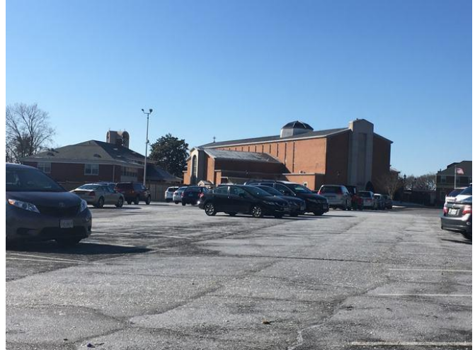
House of worship and parking lot east of the Subject
