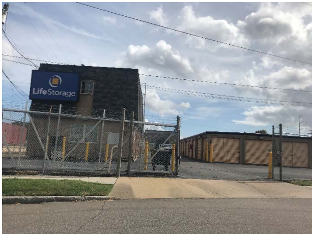
Storage facility east of Subject site
