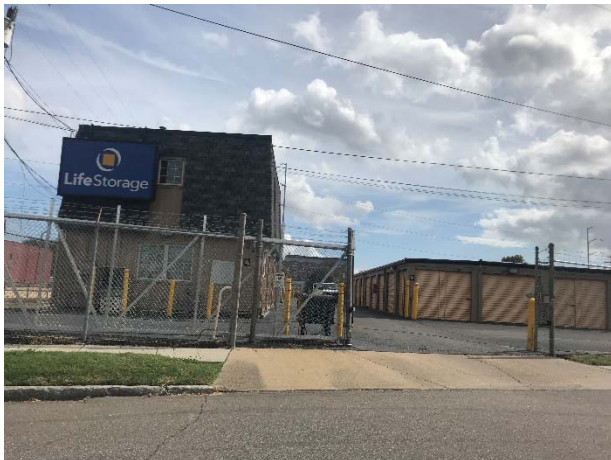
Storage facility east of Subject site
