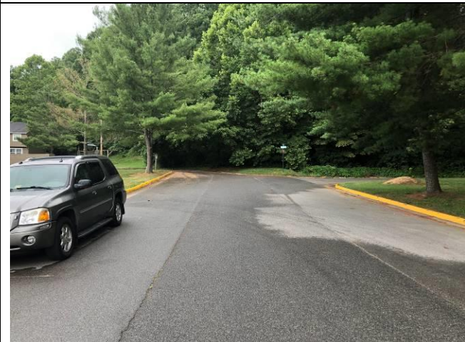
VIEW SOUTH ON FAIRFAX STREET
