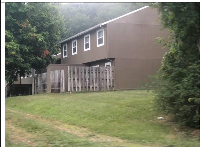
SUBJECT EXTERIOR AND FENCED PATIO
