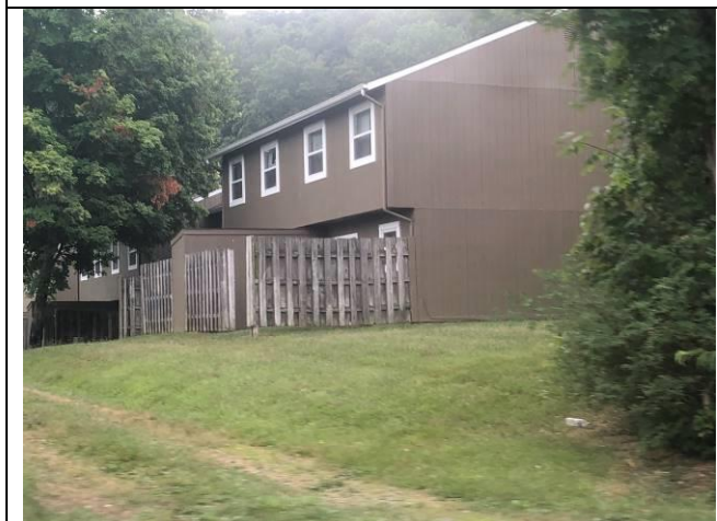
SUBJECT EXTERIOR AND FENCED PATIO
